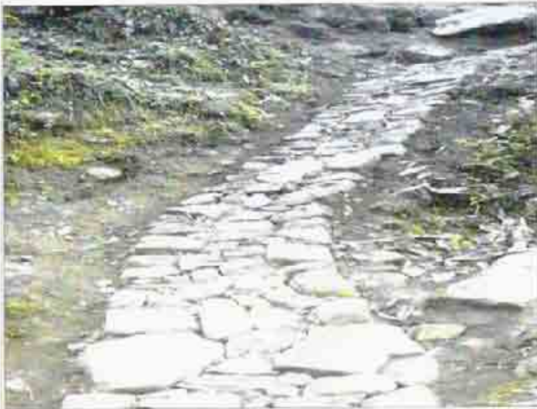
Trekking trail constructed at Chowri-Yambong 2009, in West Sikkim.
