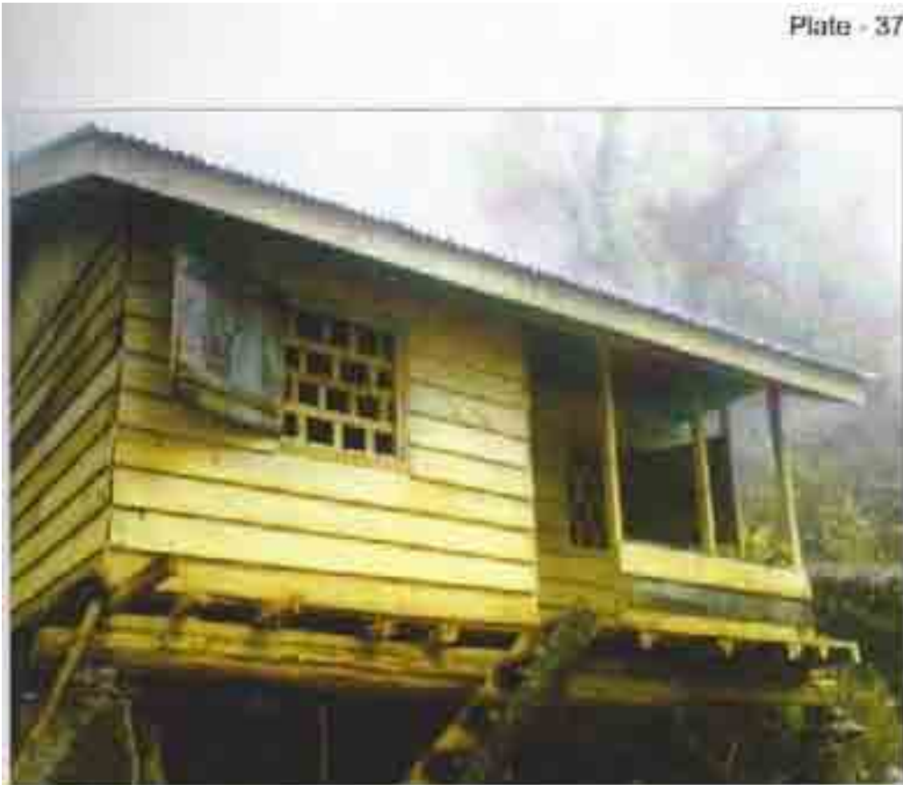
Newly Constructed Log Hut at Zali, North Sikkim.
